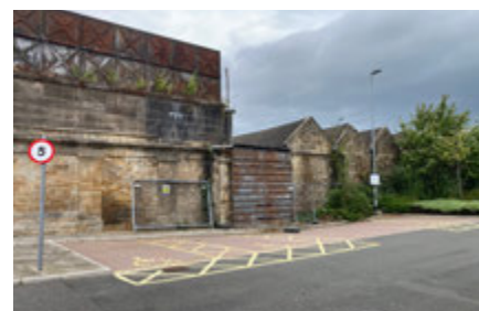
Hexham Old Goods Shed and Water Tower
