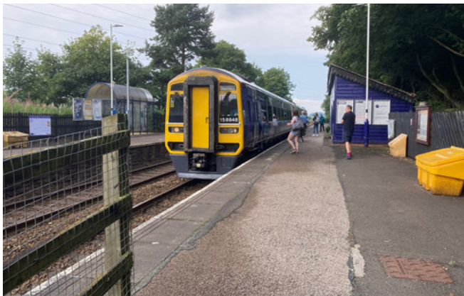
Lack of tactile paving
